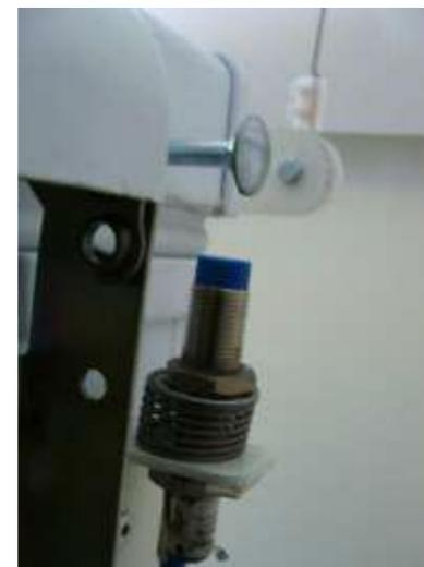
Fig. 1.4 c Sensor of "freezer opened" (machine rear)
